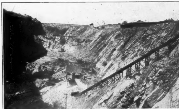
Quarry and Incline to Plant
